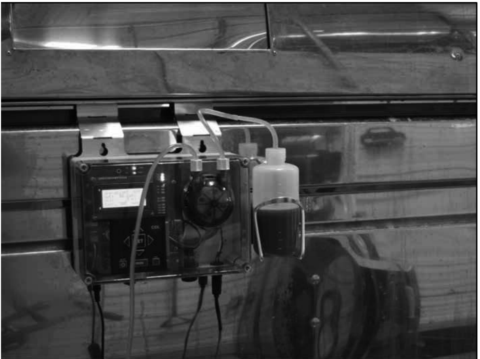
Automatic defoamer dispenser (probe not shown).
