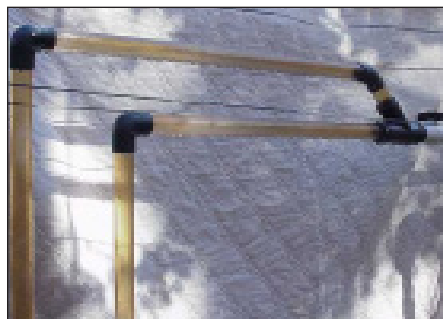
Top Portion of Two Pipe Lift
