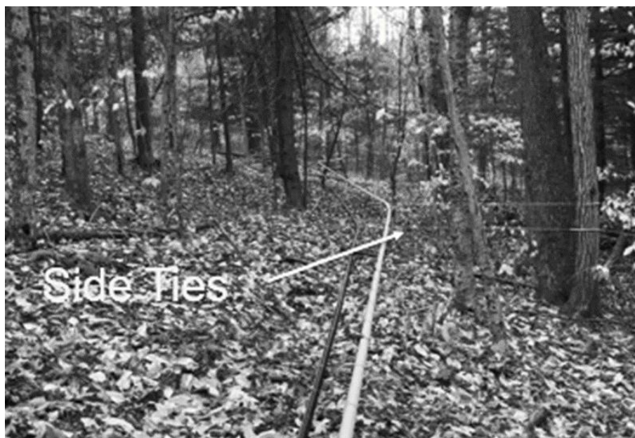
If possible, side tie to a strong, healthy tree of low commercial value, such as ironwood.
