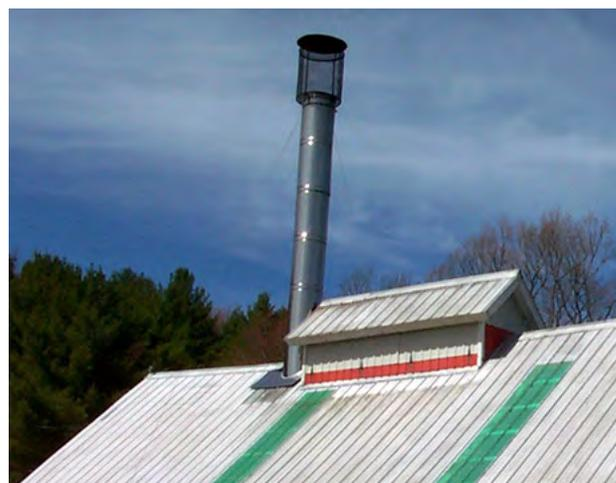
**FIGURE 7.7.** A spark arrestor is useful in preventing release of these potential fire starters.
