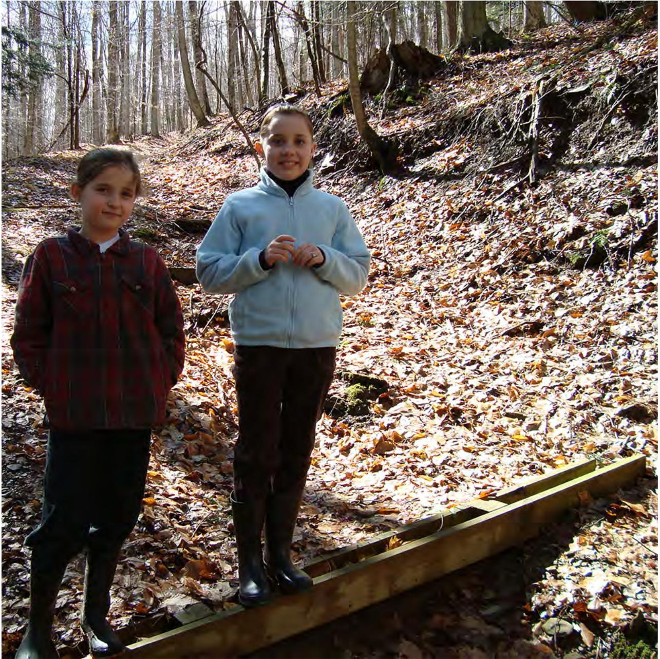
**FIGURE 5.33.** Failure to maintain water bars, open-top culverts and similar water control structures can damage the road or render it less functional. This open-top culvert was installed at the correct angle, but lack of maintenance allowed the road to wash out on the lower side of the culvert.
