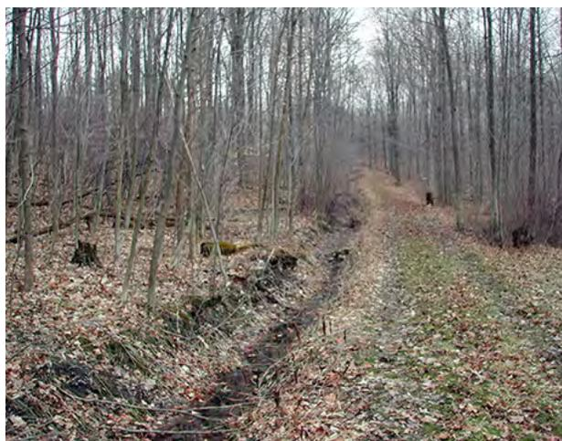
**FIGURE 5.26.** An example of an acceptable sugarbush road. The road has a ditch on the uphill side, is crowned and slightly sloped to the downhill side, and enough light is currently available to maintain vegetative cover on the road.
