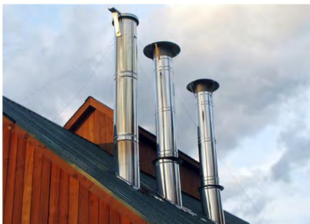
**FIGURE 12.12.** Steam stacks (two rearmost) for venting water vapor from evaporator.
