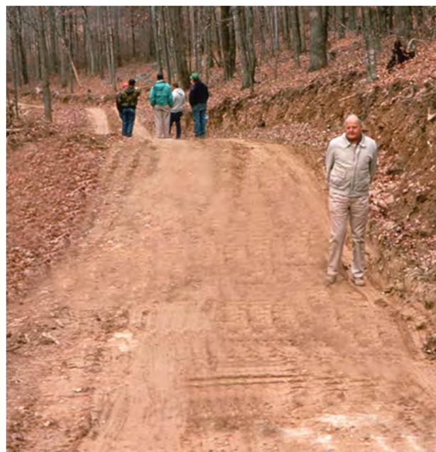
**FIGURE 5.29.** A broad-based dip (foreground) is a low, relatively flat, out-sloped diversion in the roadbed designed to intercept water flowing down the roadbed and drain it to the side, off the road surface. Note the crowned aspect to the roadbed on the rise in the background to facilitate drainage to both sides.
