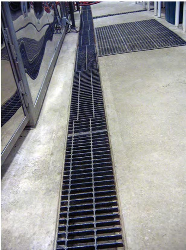
**FIGURE 12.6.** Floor drainage in the sugarhouse might include a drain running the length of the evaporator or one running around the perimeter of the evaporator and near areas of heavy water use.
