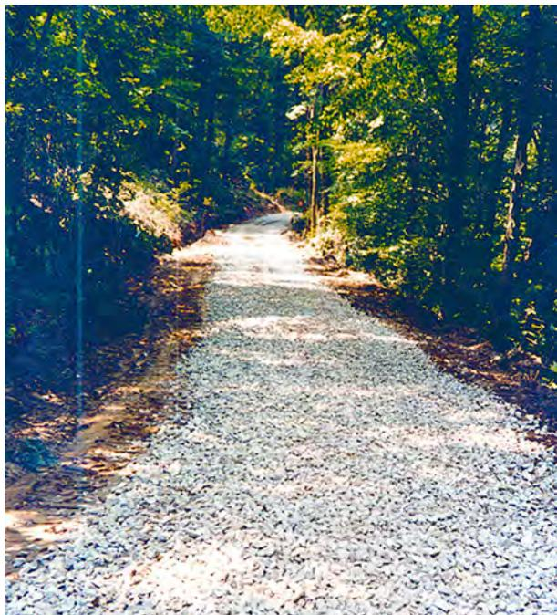
**FIGURE 5.28.** As a general rule, producers are advised to avoid developing large, heavily compacted, graveled roads in the sugarbush. Exceptions to this would be the need for a main road to the sugarhouse to support delivery or transport vehicles or customers in passenger cars. Under those circumstances, both the main road and the parking areas around the sugarhouse should be finished for access in all types of weather and conditions.”
