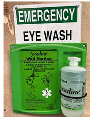
**FIGURE 13.7.** Portable eye wash station suitable for heated spaces (RO room) can be placed in the sugarhouse where chemicals are used.
