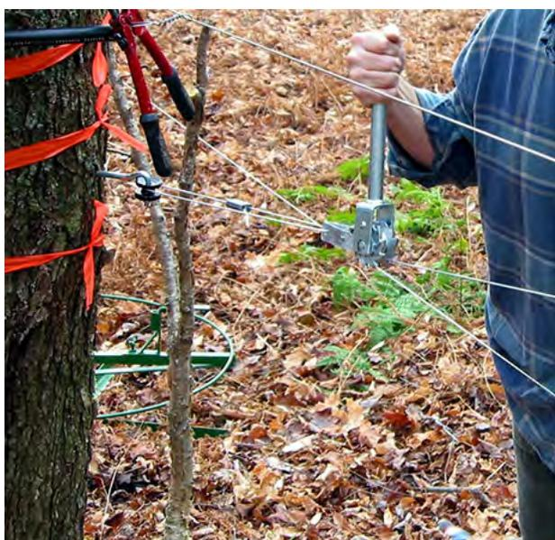
**FIGURE 6.20.** Tightening mainline support wire with a fence wire tensioner
