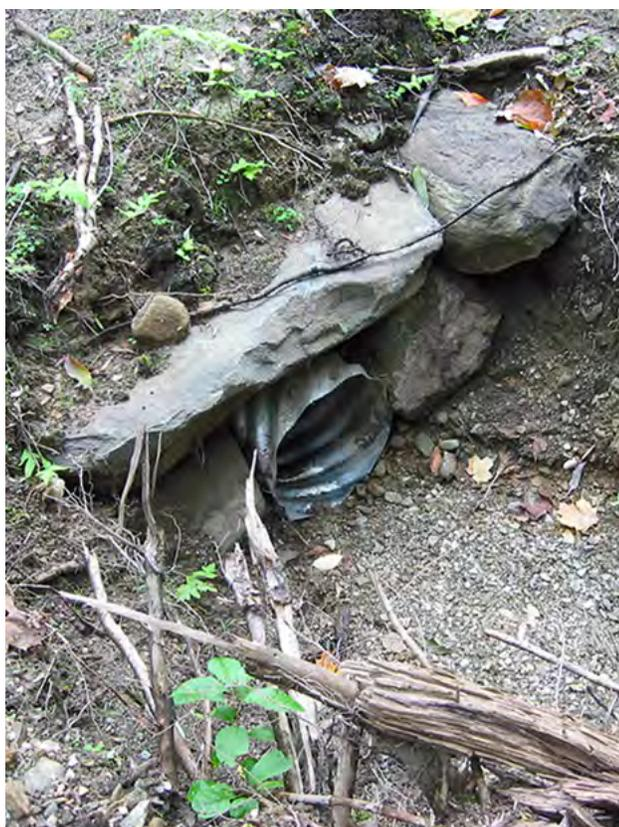
**FIGURE 5.32.** Closed culverts are conduits that move water from one side of the road to the other without it flowing across the road surface. A closed culvert would be used, for example, to move water from a drainage ditch on the up-slope side of a road to the downslope side.
