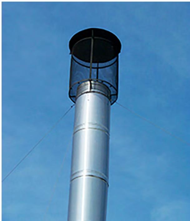
**FIGURE 13.8.** A spark arrester on top of smokestack will help reduce the chance of accidental fires.
