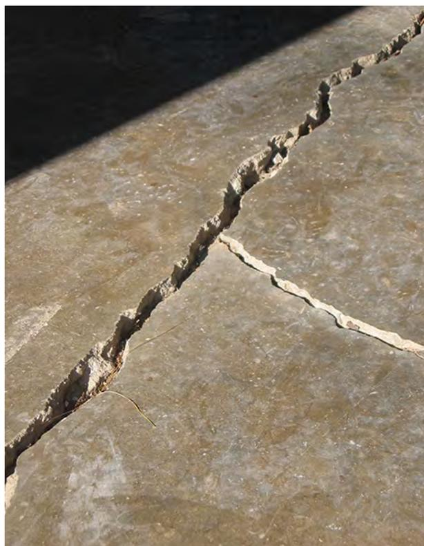
**FIGURE 12.5.** Pouring concrete on an inadequately prepared base can result in cracking.
