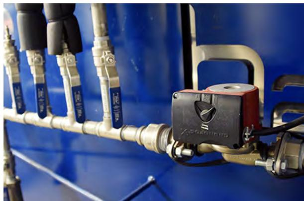
**FIGURE 12.9.** Circulation pumps can be used to deliver water from storage tanks to where it is needed in unheated spaces as long as lines are drained before freezing weather.
