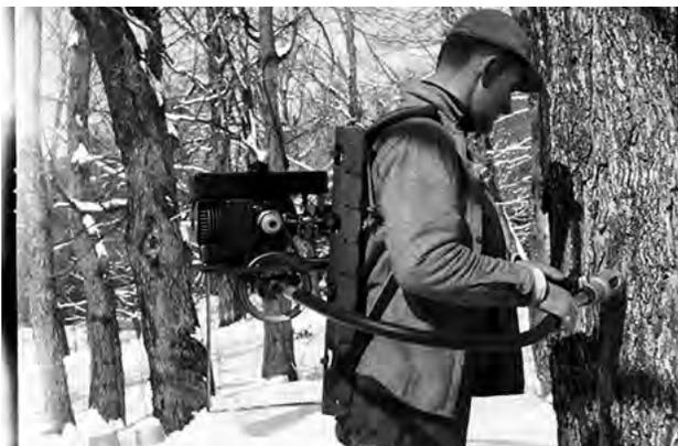
**FIGURE 2.4.** Gasoline powered tapper. (UVM LIBRARY SPECIAL COLLECTIONS)
