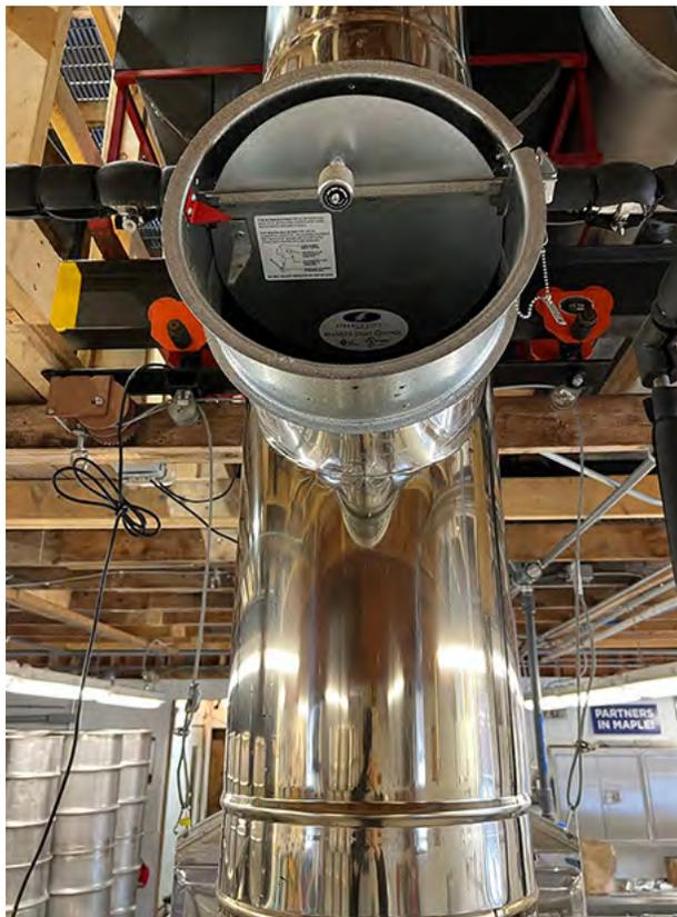
**FIGURE 7.15.** A damper is used to regulate draft. These come in mechanical or automatic styles.
