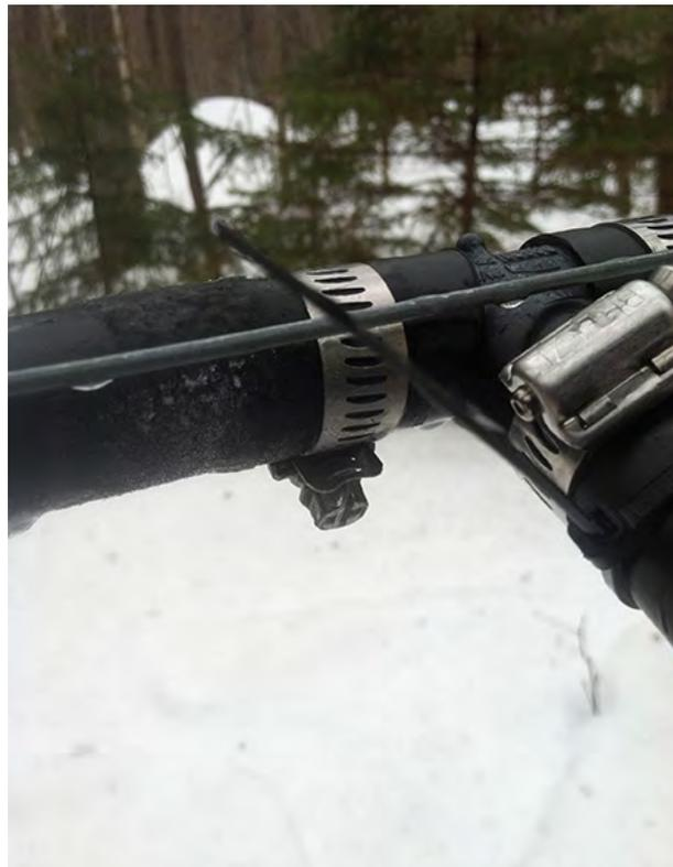
**FIGURE 6.38.** Transitory intermittent ice formation (frost on mainline to the left of the band clamp) caused by microleaks can occur in mainline systems at above freezing temperatures. This leads to loss of vacuum in sections of the woods until the frozen section thaws. These types of leaks are extremely difficult to find and correct.
