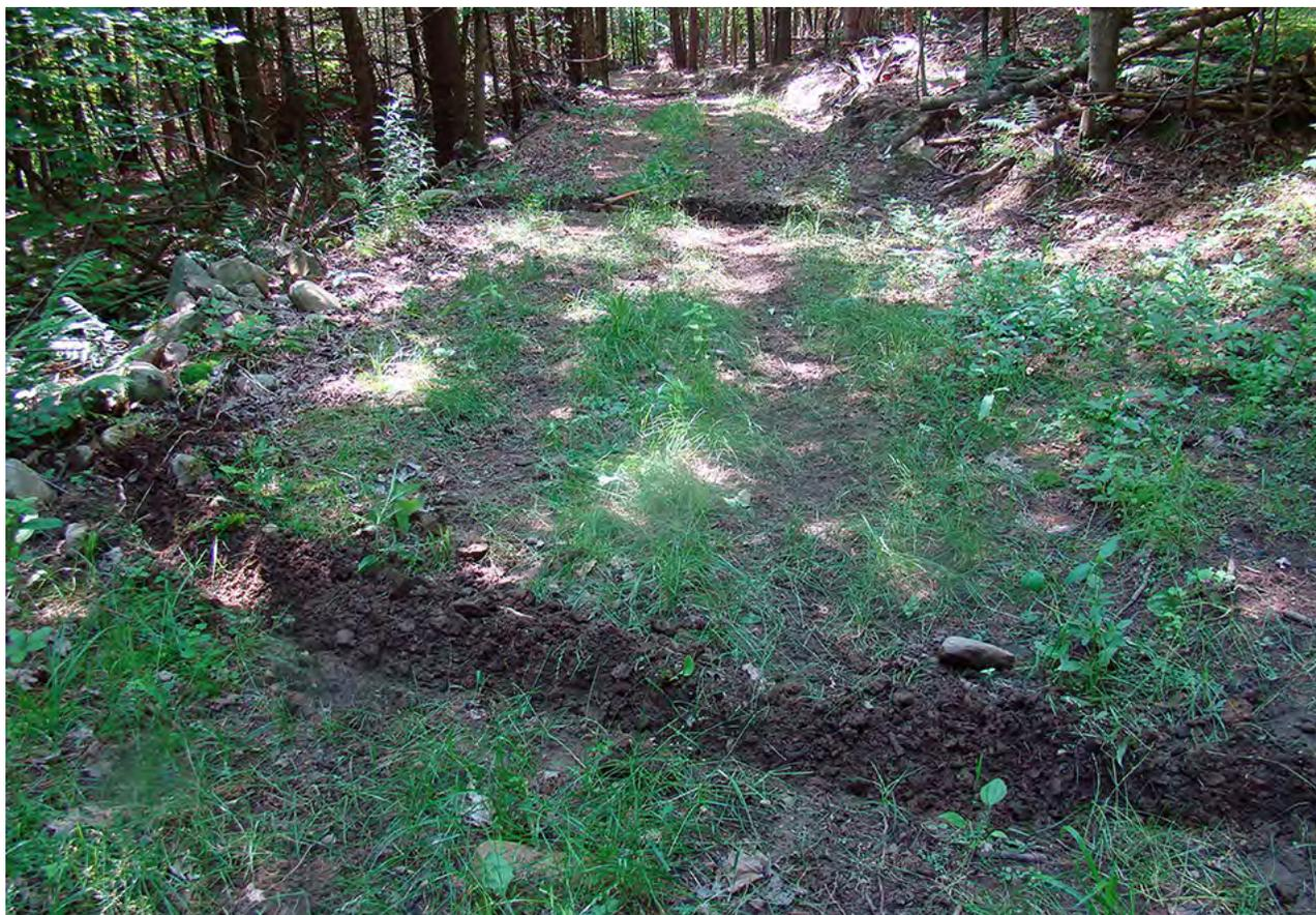
**FIGURE 5.30.** Hand-dug water bars on this low-use ATV trails are oriented approximately 30 degrees to the downhill side. Spacing depends on the steepness of the slope of the trail.
