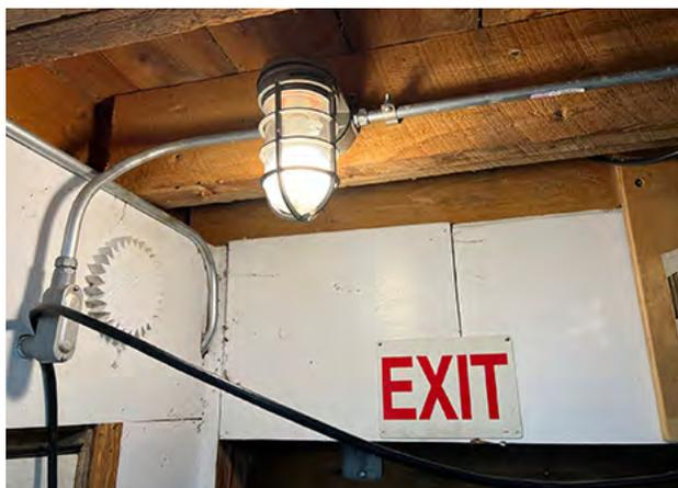
**FIGURE 13.10.** All lights in areas where sap is stored or syrup is processed should be shielded to prevent breakage and glass entering the product.
