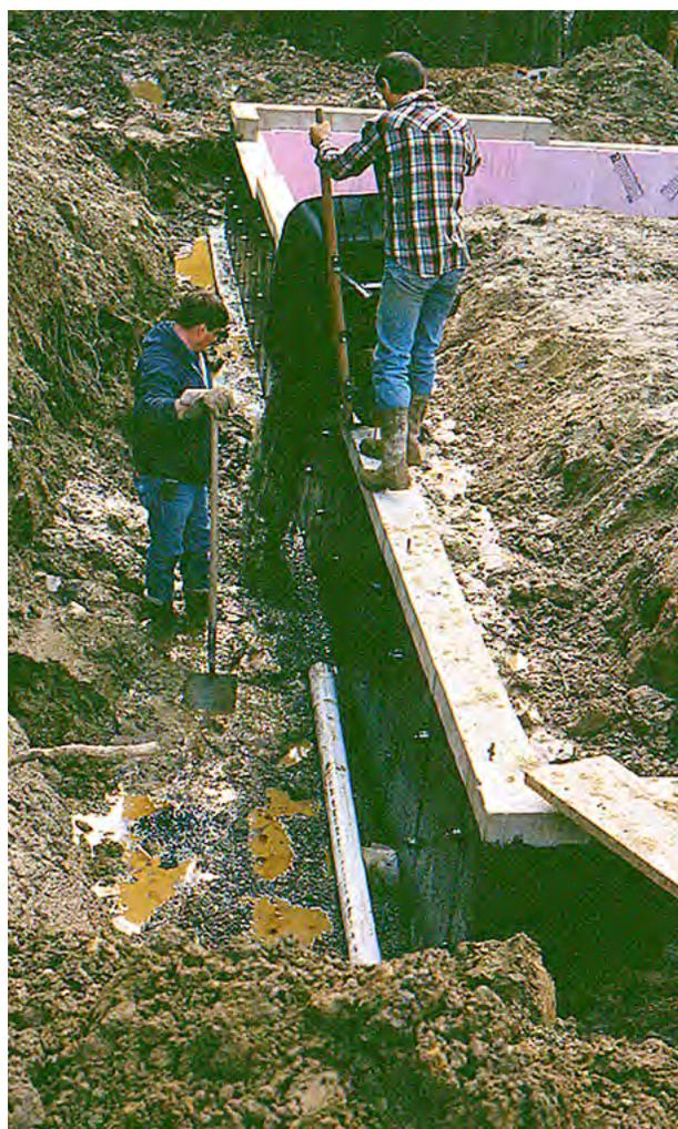
**FIGURE 12.4.** Sugarhouses are often built in low-lying areas. Increasing the amount of gravel and adding perforated pipe and curtain drains to control ground and surface moisture will help prevent frost damage to the foundation.
