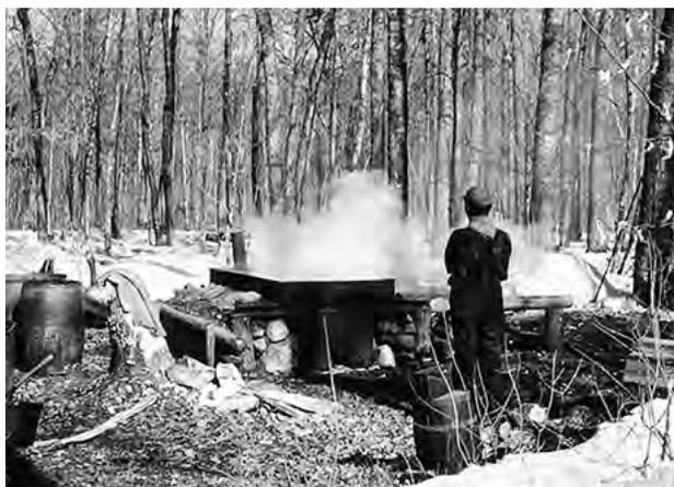
**FIGURE 2.11.** Boiling outdoors on a flat pan setting on a stone arch.
