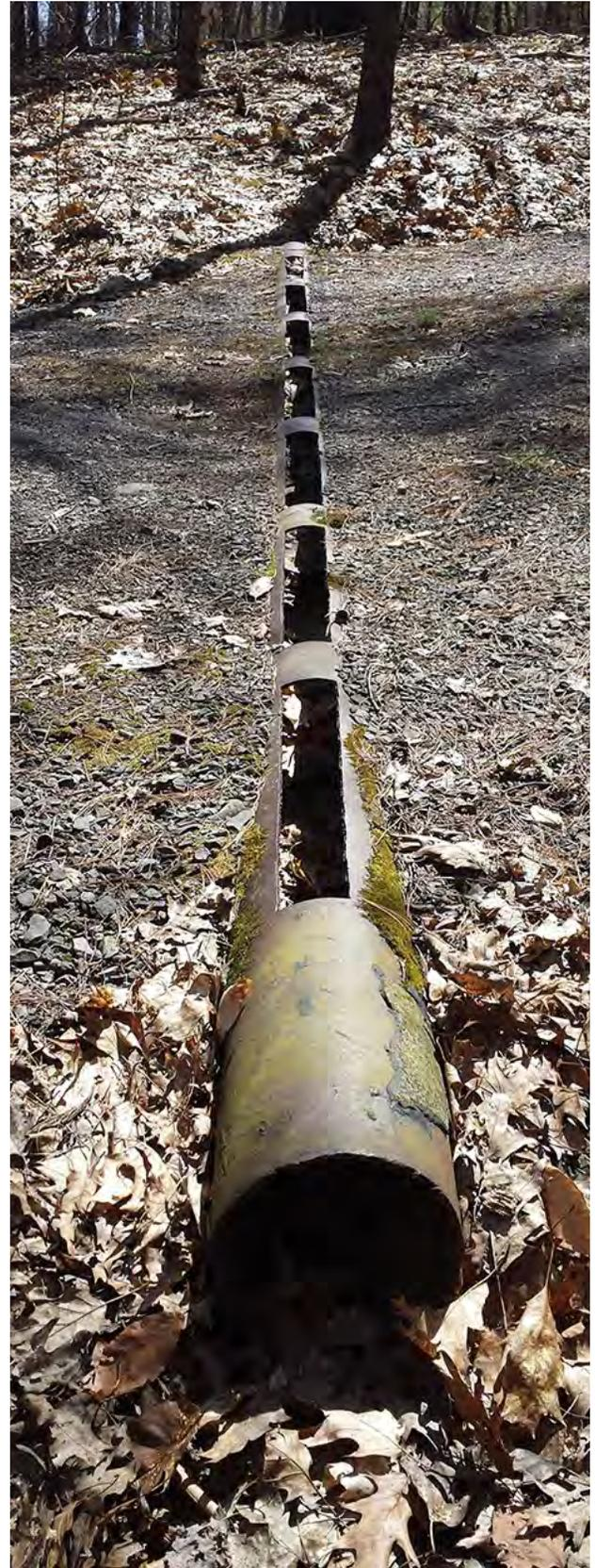
**FIGURE 5.31.** Two examples of open-top culverts. These are installed at a down-slope angle across a road or trail to intercept water and carry it off the road. Culverts require regular maintenance to clear debris.
