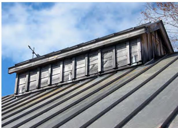
**FIGURE 12.13.** Cupola with pulley system to vent steam from sugarhouse.
