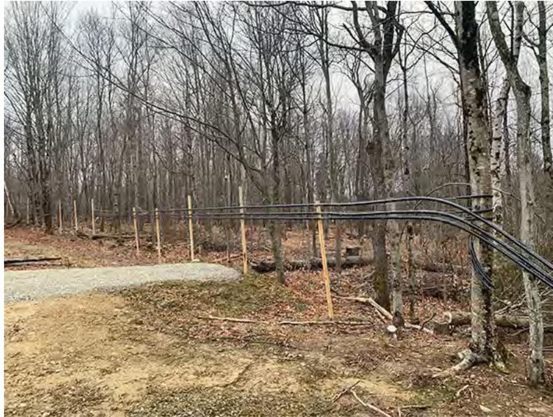
**FIGURE 6.18.** Standard maple mainline supported on wire and kept in position with posts. The three lines represent wet and dry conductor lines and a pump line.
