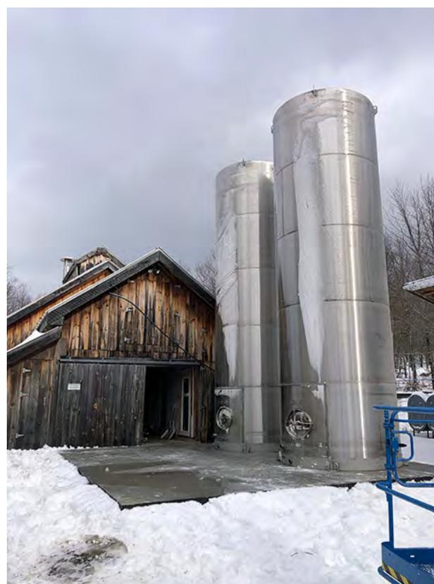
**FIGURE 6.43.** Transfer and storage tanks for sap come in a wide variety of sizes and configurations and should be food-grade, clean, and suitable for intended use.
