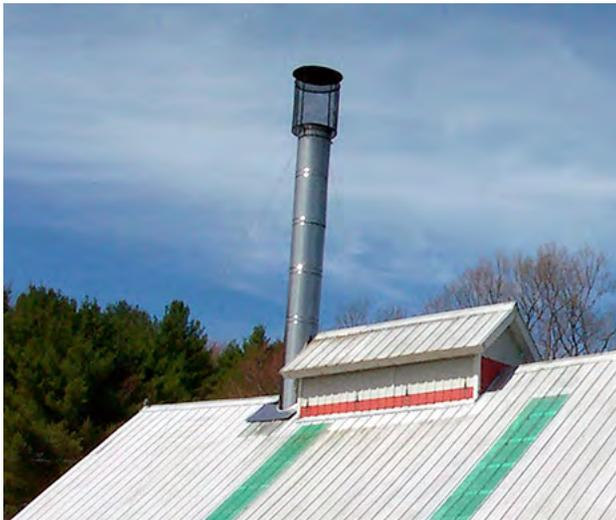
**FIGURE 12.14.** A spark arrester is useful in preventing release of these potential fire starters.
