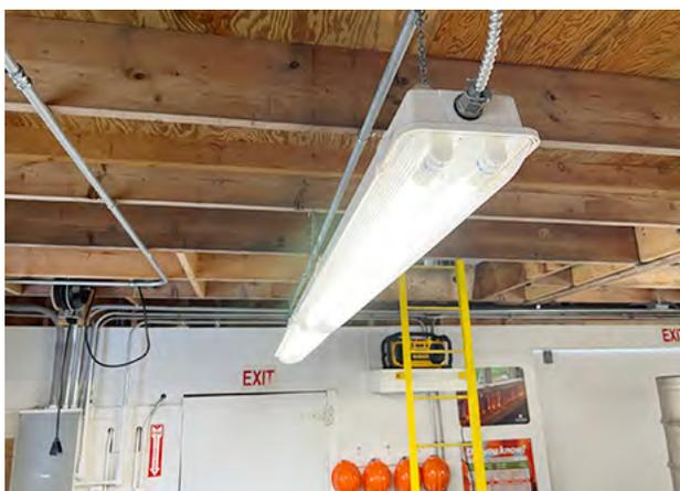
**FIGURE 14.3.** Light fixtures in facilities producing or packaging maple syrup should be properly shielded to prevent accidental contamination of syrup if bulbs are broken.
