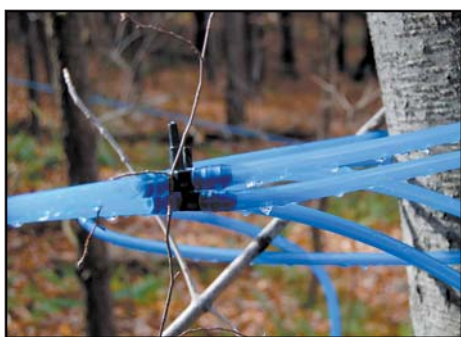
New 3/16ths tubing can be worked into existing mainline systems.
