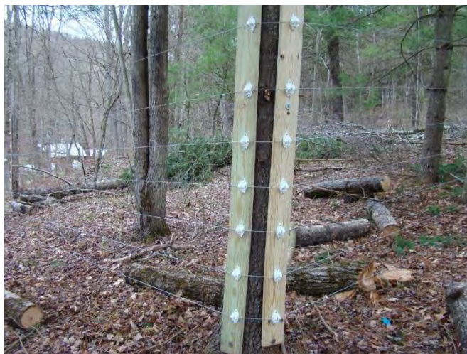
Figure 16. On abrupt corners, double batten boards may be necessary to protect the tree. Abrupt corners increase resistance when pulling wire around perimeter.
