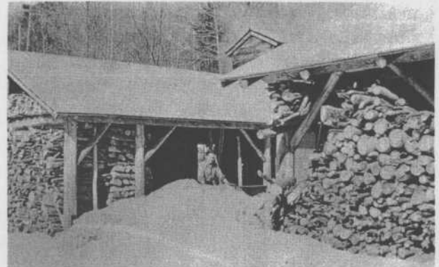
Figure 4. Open-sided wood storage.
