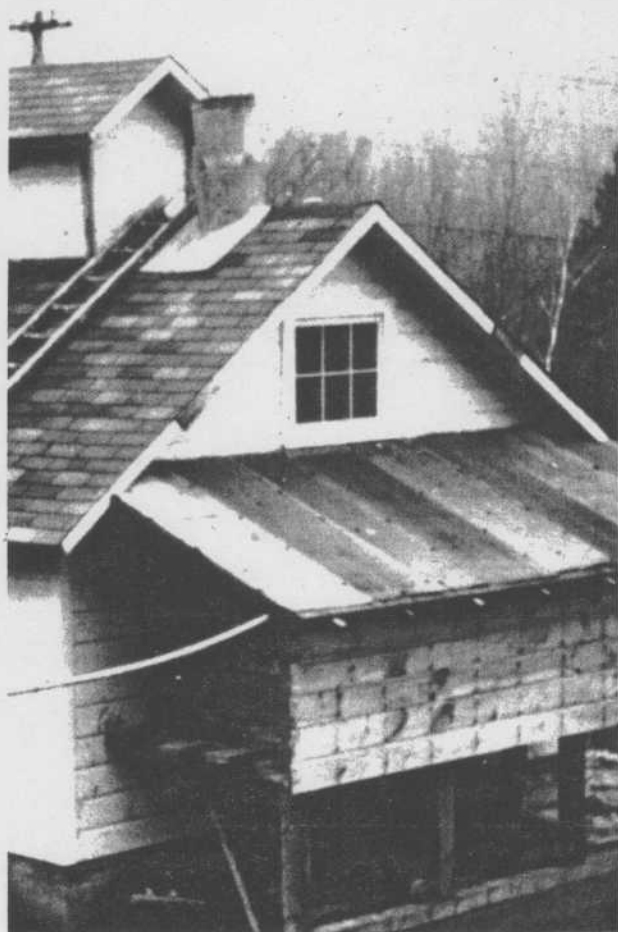
Figure 6. Sap storage located on north end of sugarhouse. Note gravity feed line.
