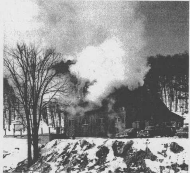
Figure 2. Sugarhouse located for good draft and air drainage.
